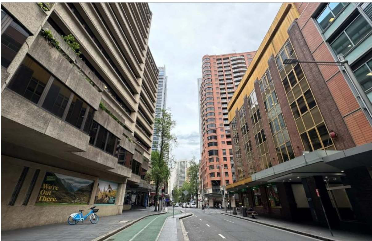
Figure 6: View of Kent Street, facing south
